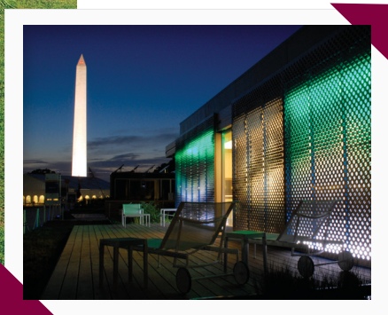
A BRIGHTER WAY: LumenHAUS now resides on the Blacksburg campus adjacent to Cowgill Hall. (top right) Open house of LumenHAUS, 2011. (middle right) LumenHAUS 2010. (bottom right) On the Washington, D.C., Mall at the 2009 Solar Decathlon.
